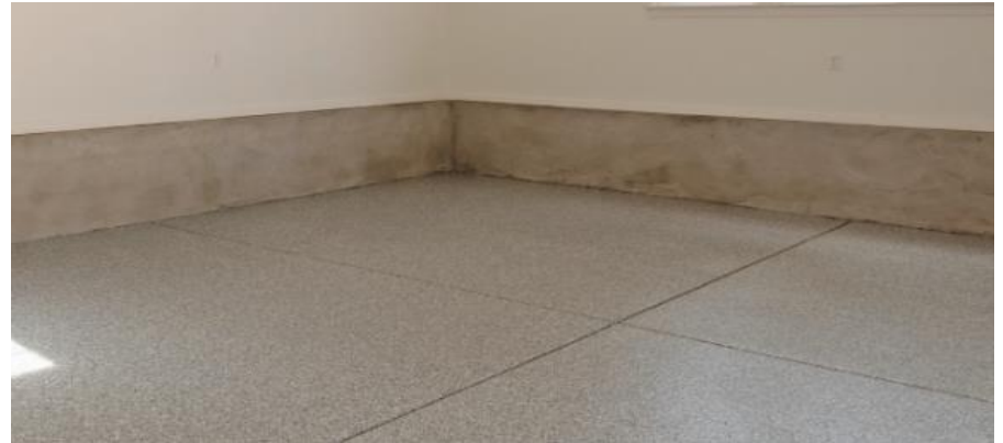
Epoxy Garage Floor Coating
