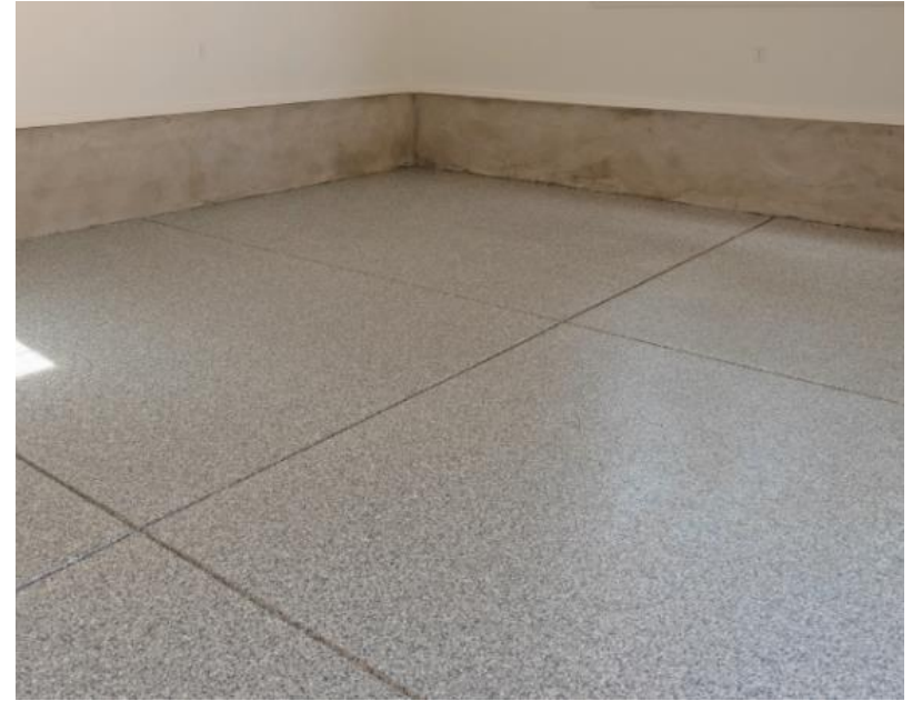
Epoxy Coating at Garage Floor
