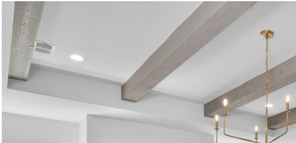
Cedar Ceiling Beams at Foyer x4
