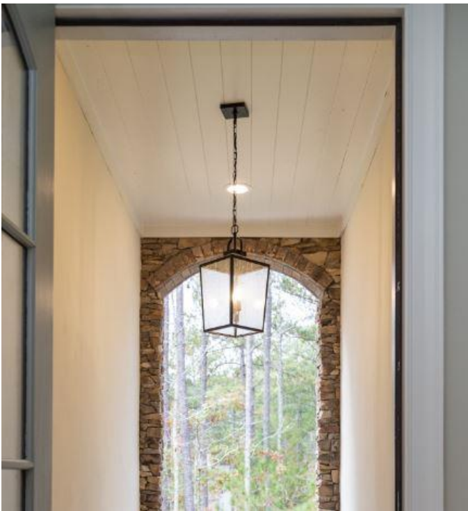
Tongue & Groove Ceiling Detail
