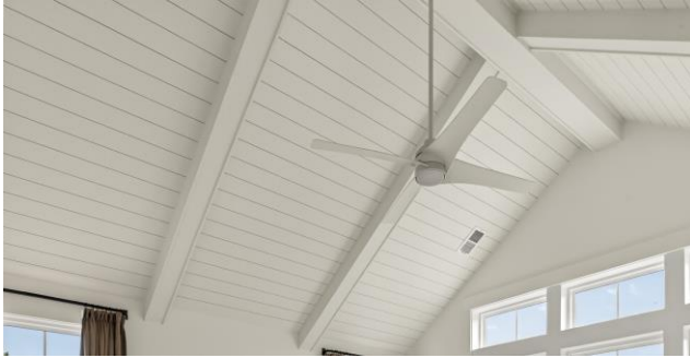
VERTICAL 1X4 BATTENS W/ SQUARE GROOVE CEILING & BEAMS
