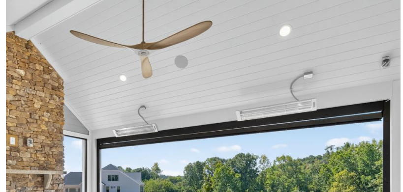
Tongue & Groove Ceiling Detail: Covered Outdoor Living & Front Porch
