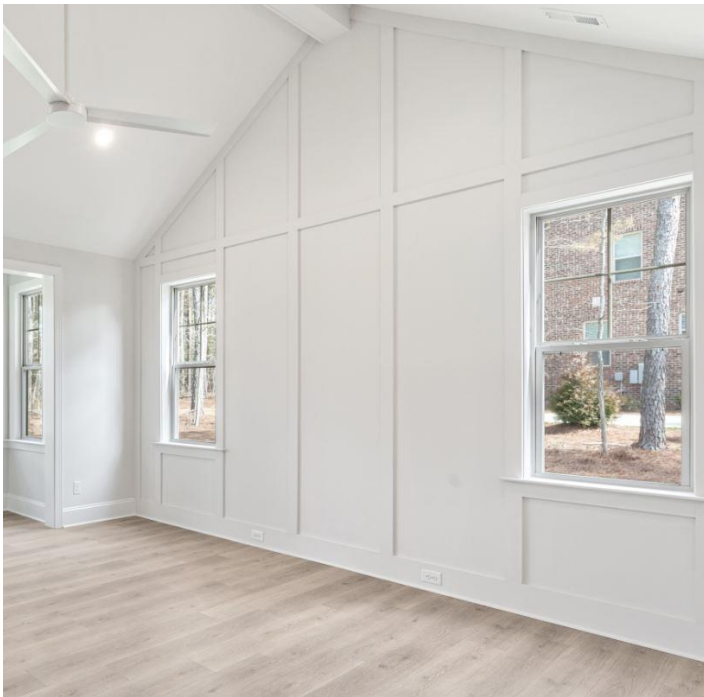
VERTICAL 1X4 BATTENS W/ SQUARE GROOVE CEILING & BEAMS
