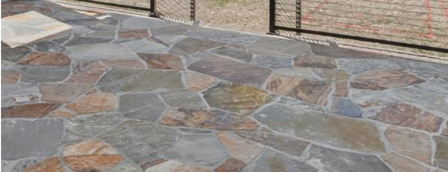
Flagstone Pavers: Front Porch & Covered Outdoor Living
