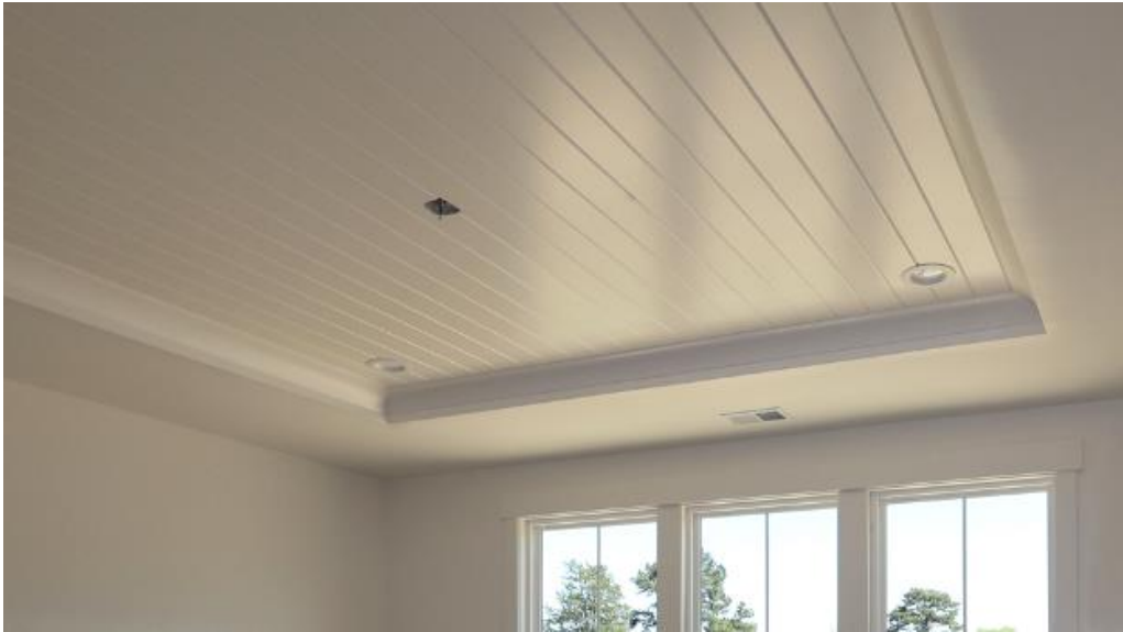
Dining Room Tray Ceiling
