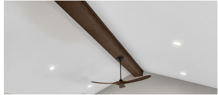
Cedar Ceiling Beam
