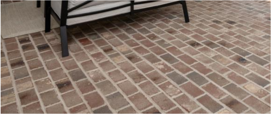
Brick Paver *Also at Basement Patio
