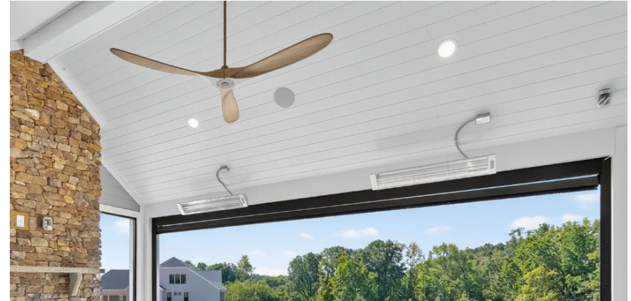
Tongue & Groove Ceiling Detail
