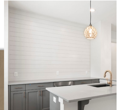
Shiplap Wall Detail
