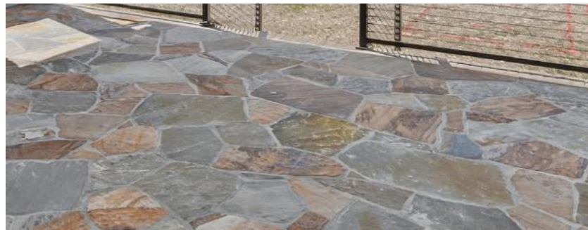
Flagstone Pavers: Front Porch & Covered Outdoor Living
