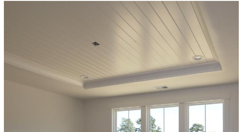
Inside Tray Ceiling
