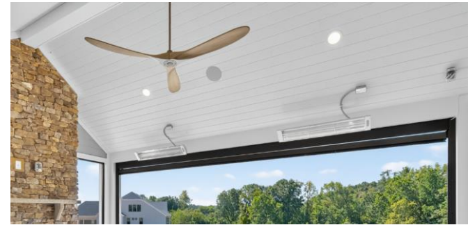
Tongue & Groove Ceiling Detail
